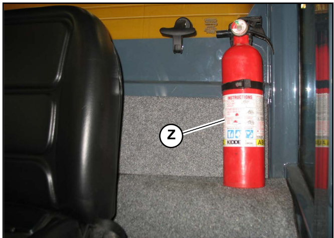
Fig. 3 – Location for Fire Extinguisher
