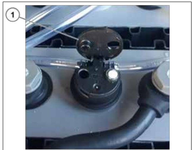
Figure 81: Checking the density of the electrolyte in the high-voltage batteries
