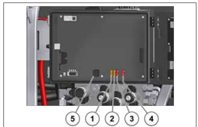
Figure 160: Replacing the ground-level control panel fuses and relays
