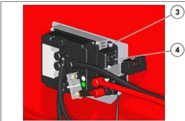
Figure 121: Cleaning the heat sinks and the wheel motor drive fans
