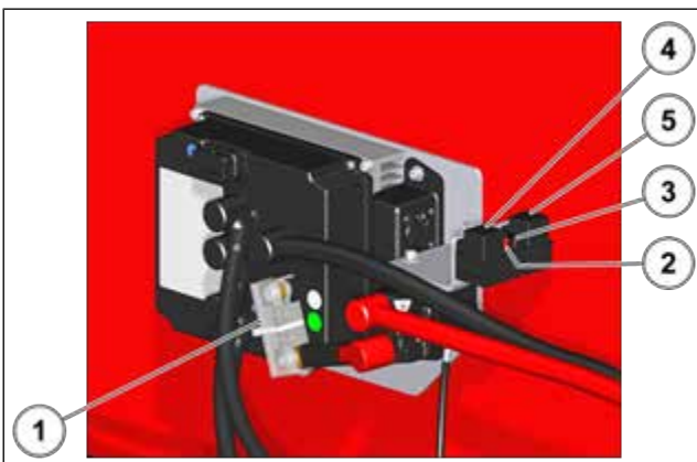
Figure 159: Replacing the wheel motor drive fuses and relays
